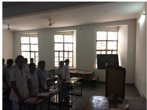
Picture 1. Poor lighting in class room
